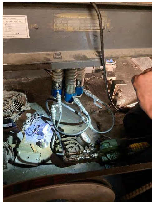
Figure 11: A hydraulic rope tension equalizer in use
