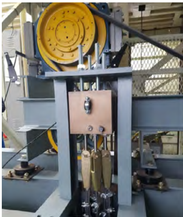
Figure 12: A permanently installed hydraulic rope tension equalizing device
