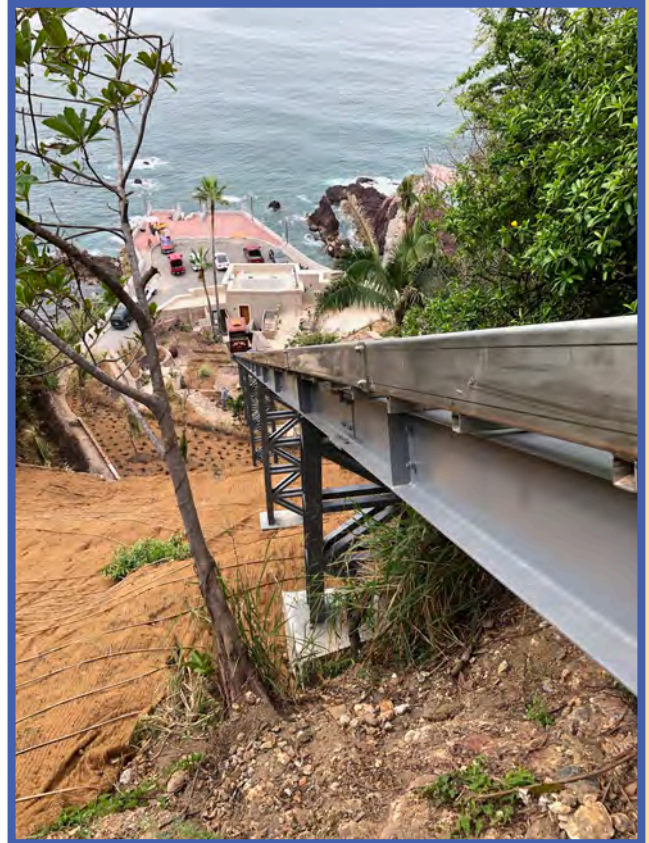
The elevator traverses the steep hill.
