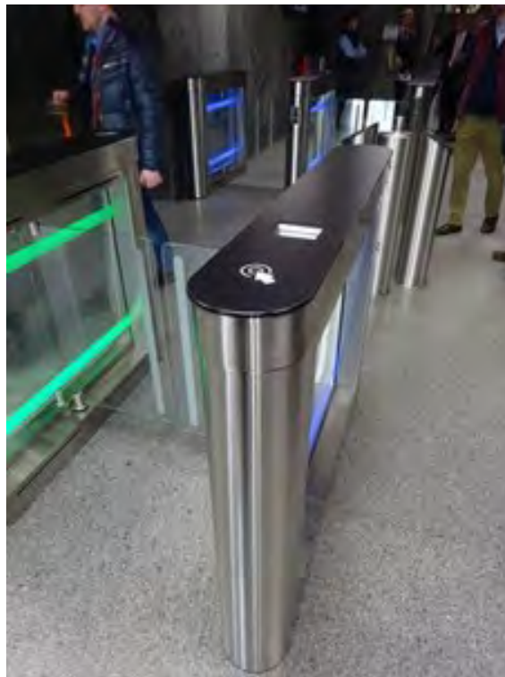
A Resuelve building access system that includes smartphone operation
