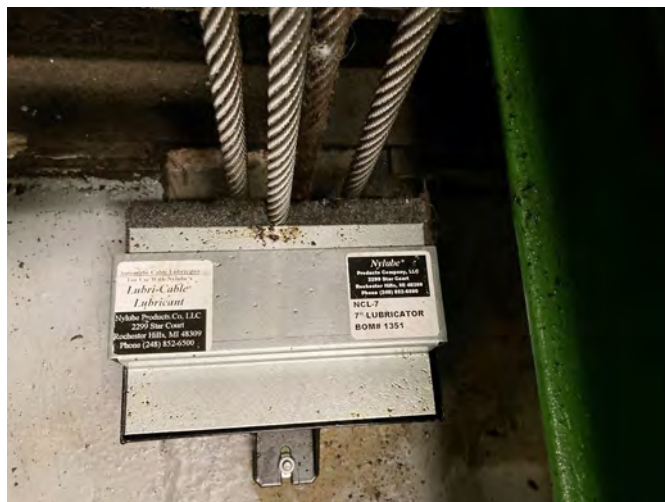
Figure 14: automatic rope lubrication system
