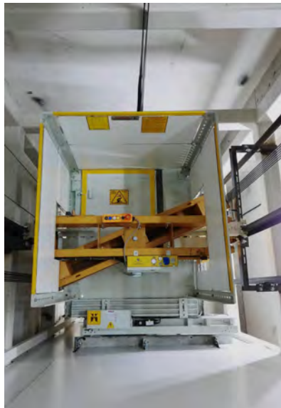
Safety gear installed on upper girder
