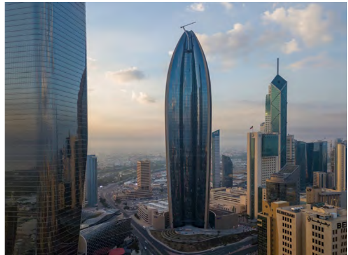
NBK's new headquarters; photo courtesy of thyssenkrupp Elevator.
