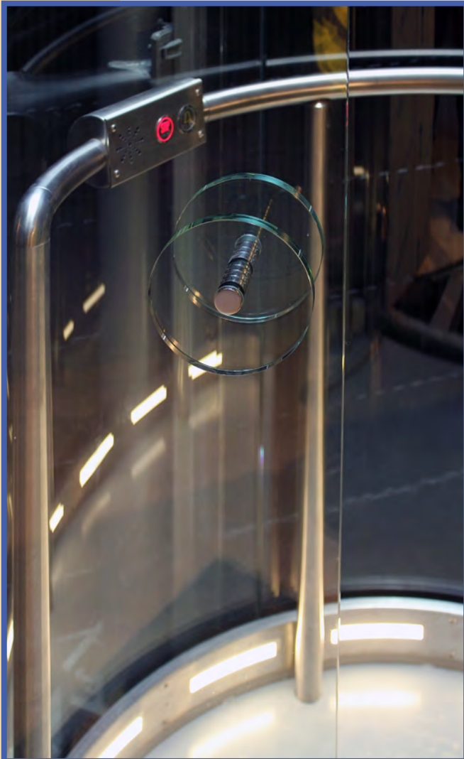
Cabin control panel/handrail
