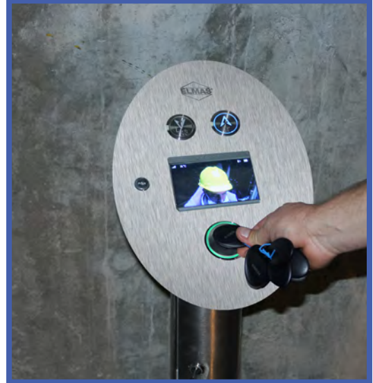
The landing operating panel is activated by card.
