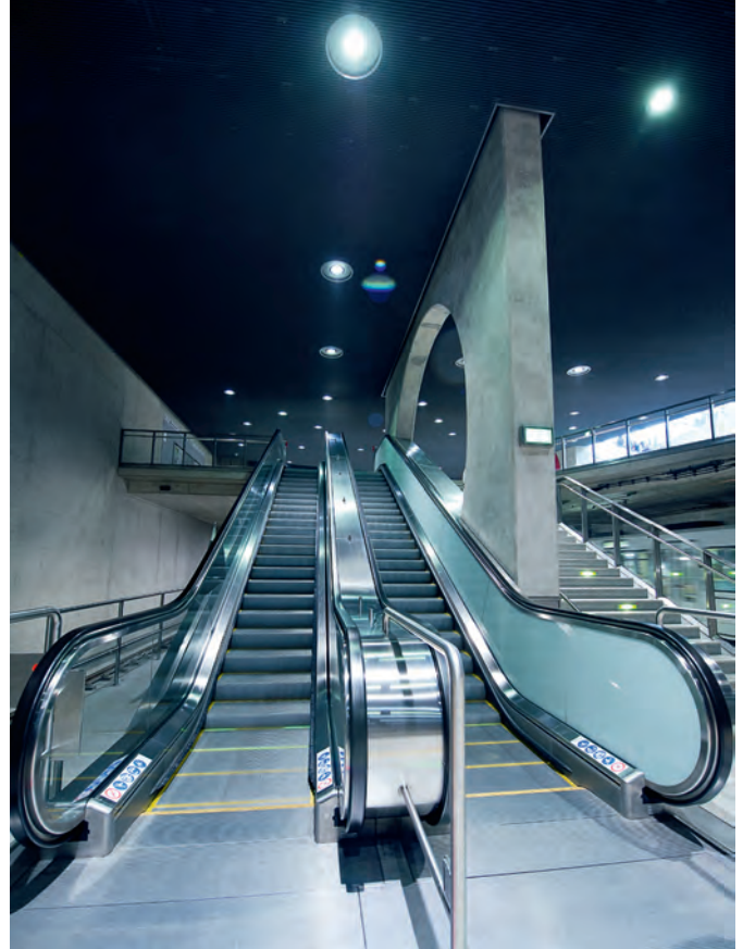
Set of heavy-duty thyssenkrupp victoria escalators serving the Ataköy-İkitelli line
