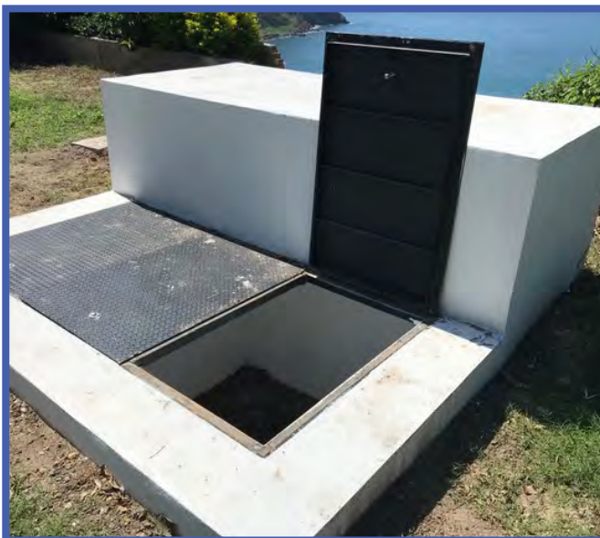
What can only be described as a concrete bunker was built to house the machine room.
