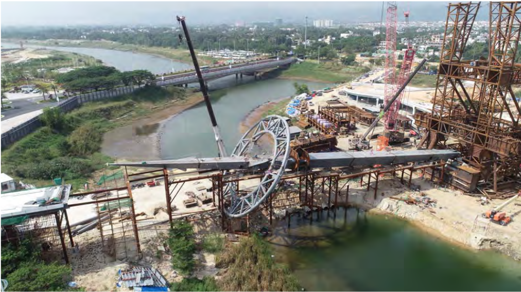
Bridge tower under construction
