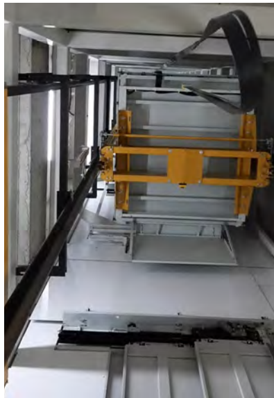
Safety gear installed on lower girder
