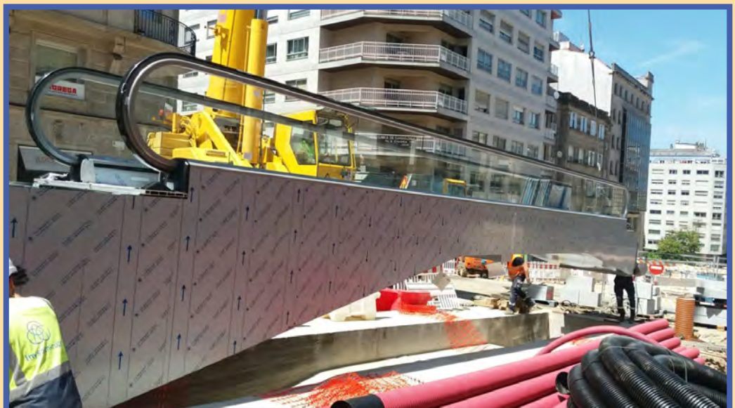
Passenger safety and comfort were prioritized to provide the streets of Vigo with light and accessibility in equal parts.
