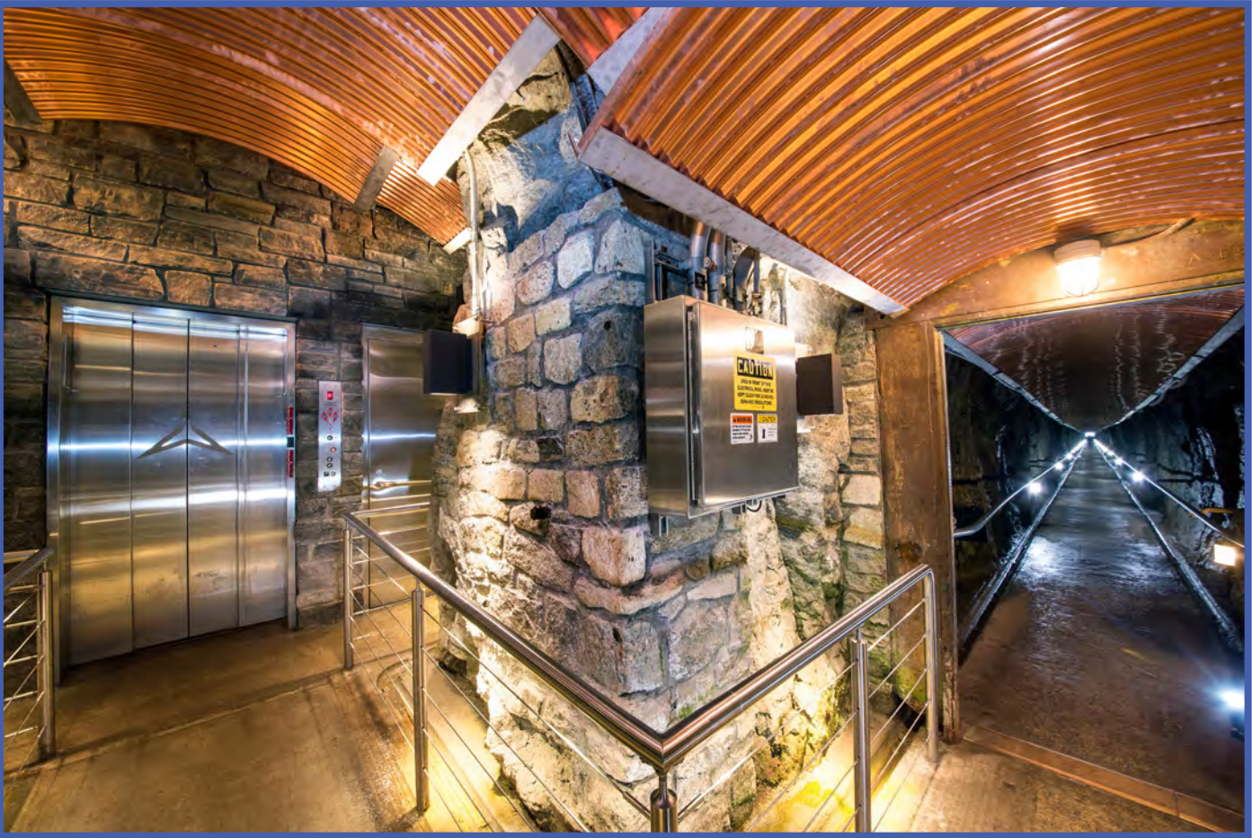
Bottom landing, at the end of the tunnel
