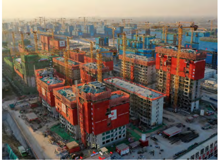
Numerous buildings are under construction in the Rongdong District of Xiong'an New Area; photo provided by Hitachi Elevator (China).
