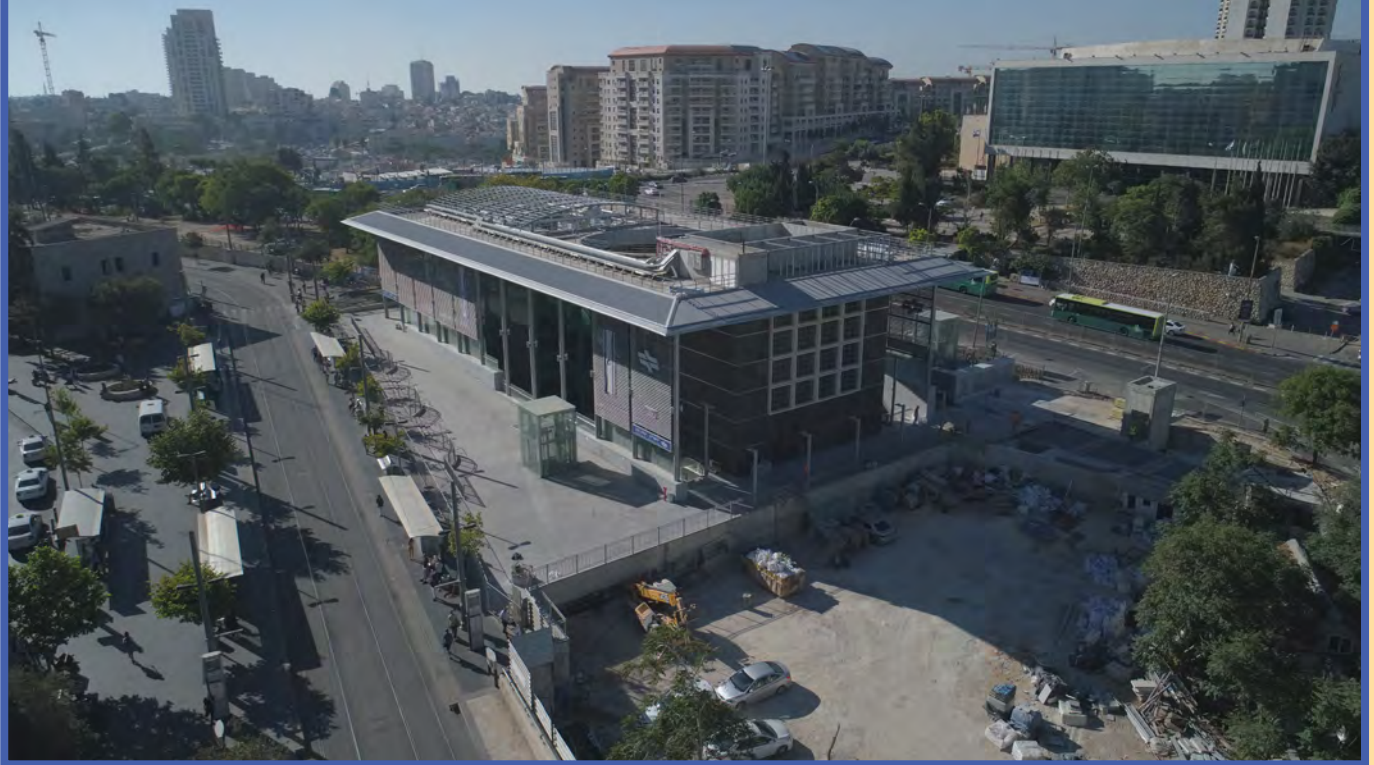
Yitzhak Navon Train Station
