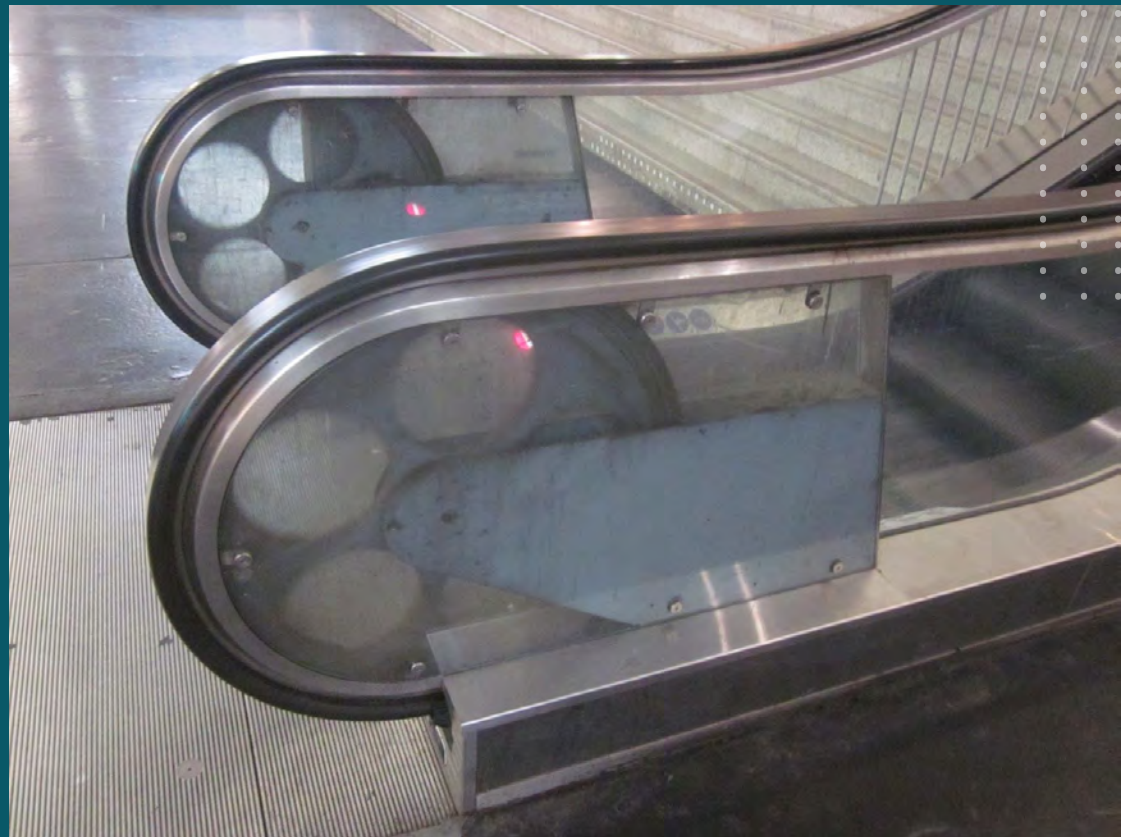
The glass balustrade with conventional handrail drive system was a design that did not find favor in the U.K.
