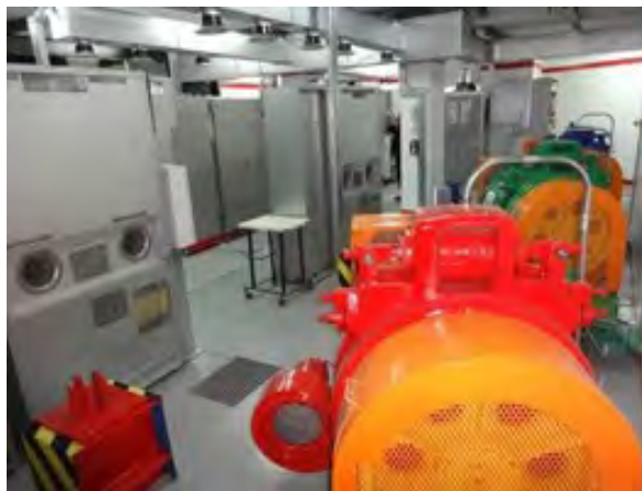
(u-d) before and after views of the machine room at Torre Europa
