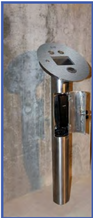
Communication system (intercom type)
