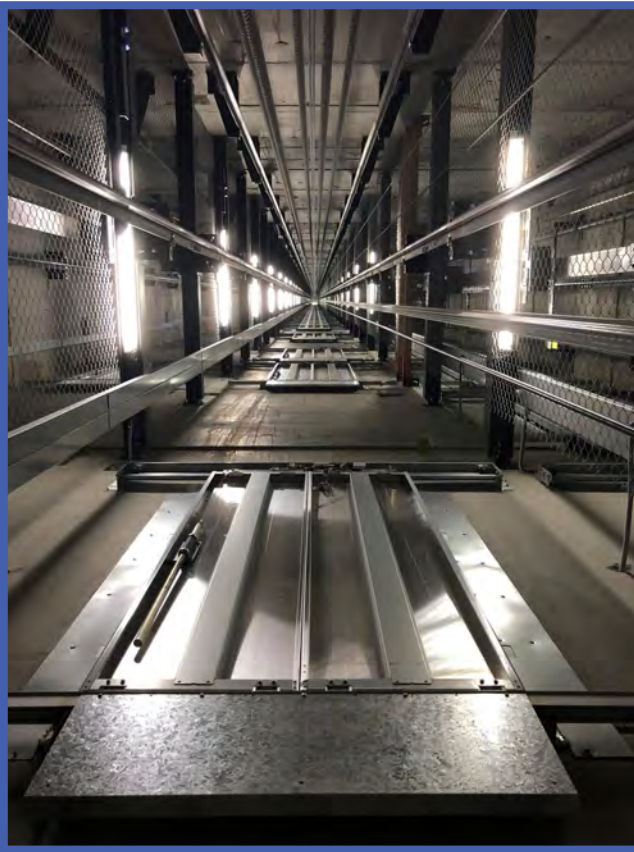
The elevator system uses a triplex arrangement for the two SkyRise elevators and the Gen2 Premier shaft, seen on the right side.
