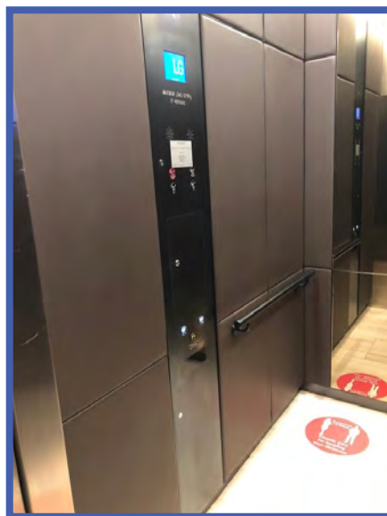
The elevator car panel lacks floor push buttons because the elevators use the Otis CompassPlus destination-management system.
