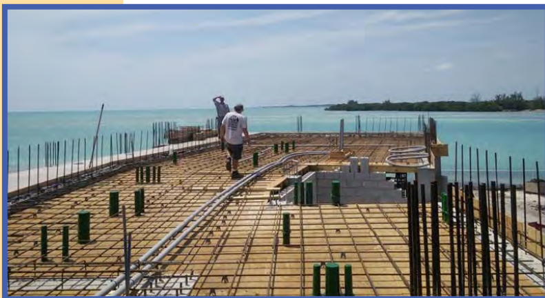
The team lays PVC pipe for elevator power cables during a site visit.
