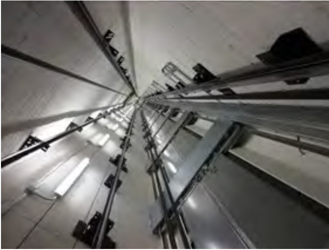
A hoistway from a Resuelve project
