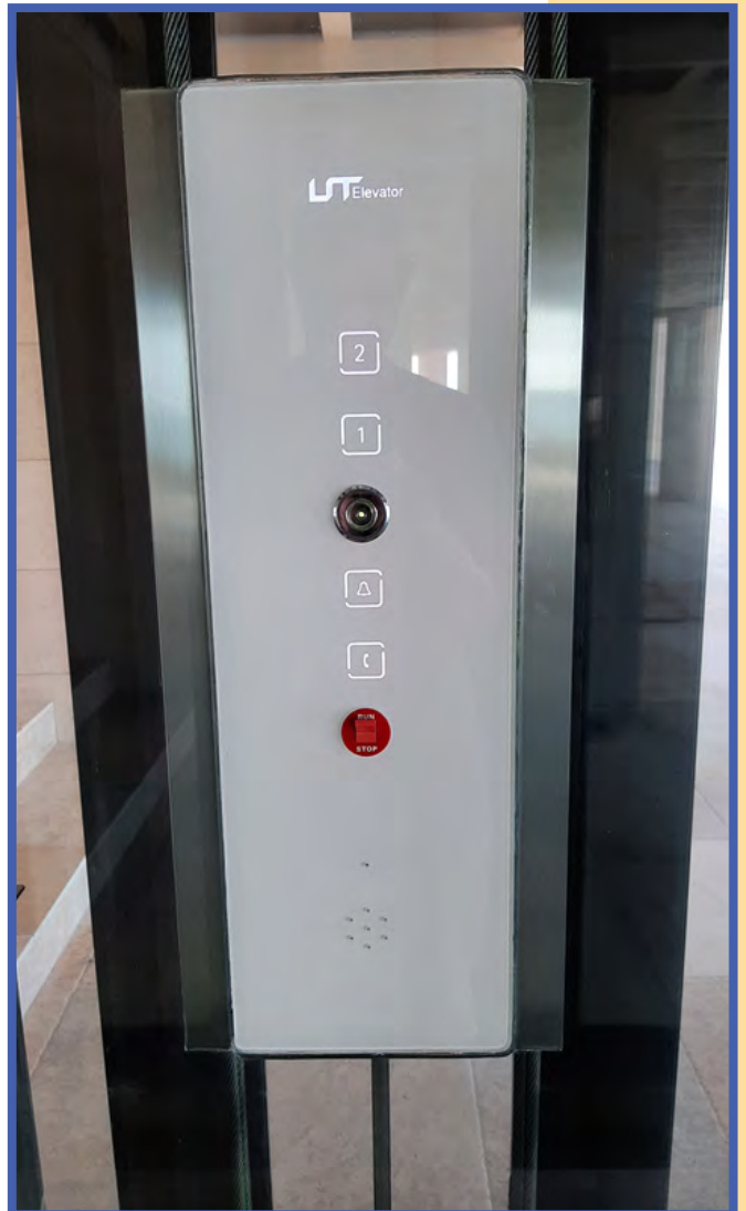
Capacitive-touch glass fixtures were embedded into the control side glass panel for a uniform, flush appearance.
