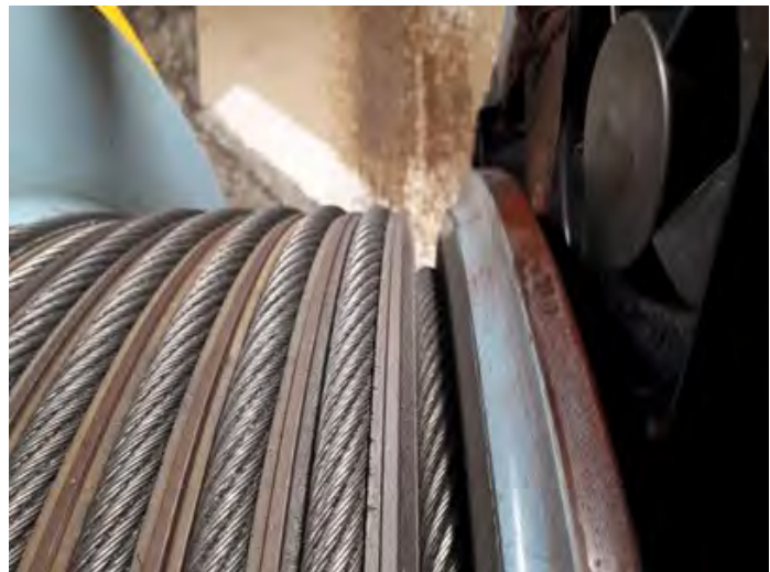
Figure 4: Excessive damage to a sheave groove
